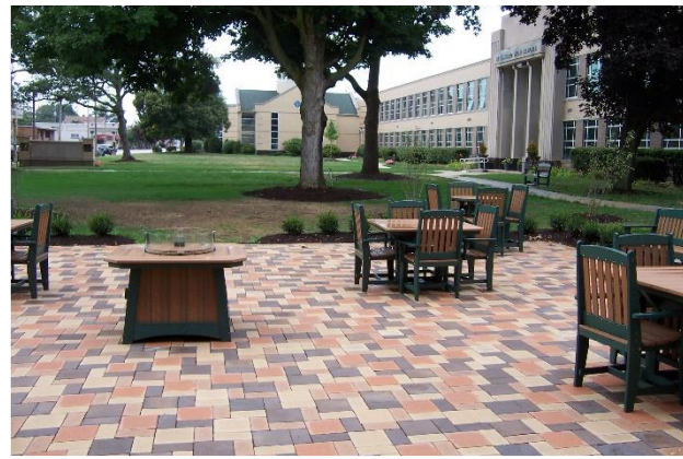
This is the view of the new patio looking south toward Detroit Avenue
