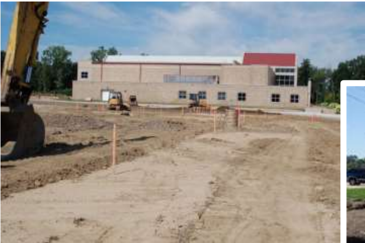
Parking Lot Construction
