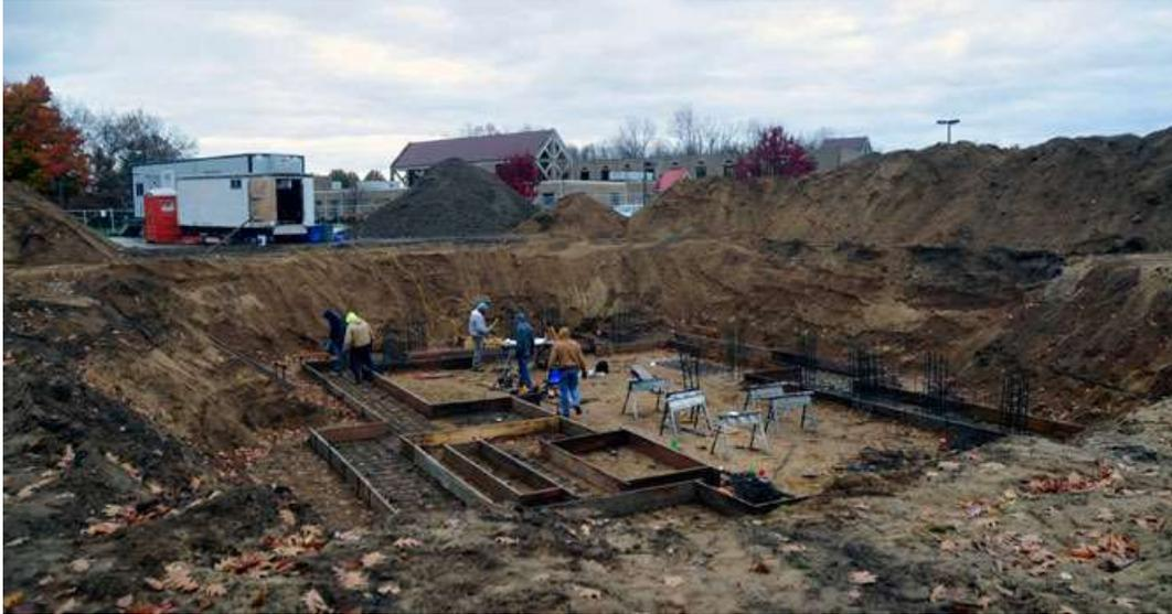
Looking at the Holy Cross College worksite it looks as though just a big hole has been dug where the tennis courts were located. A closer look into the hole will show that in the past week progress has been made building the forms which will be the foundation for the new building. In the next week or so construction work will be done in below normal temperatures. Holliday Construction of South Bend is the primary contractor on the project which will open for student residents next August.
