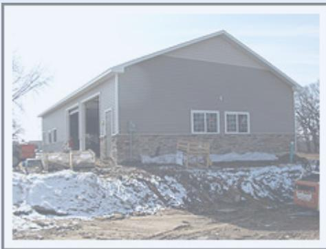
The new 4000 square foot maintenance building at Holy Cross Village is nearing completion. The shingles and siding, brickwork and doors are completed as well as the electrical systems, interior insulation and wall board. All that needs to be done is the concrete floor. The project began the first week in December. Brown and Brown is the principal contractor and the garage is built in the style of Andre Place in Holy Cross
