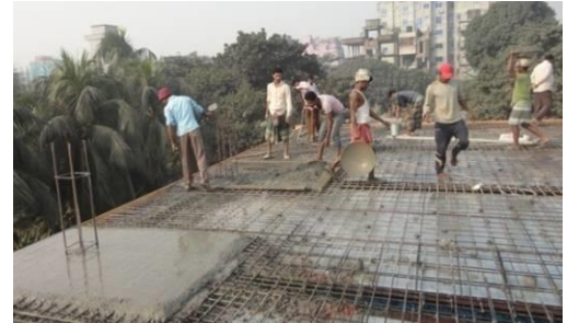
The construction of fourth floor is underway
