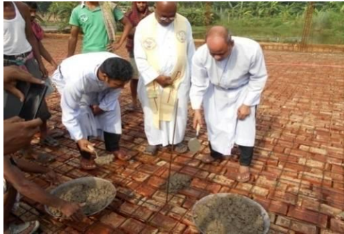
Inaugurating pouring of the basketball field
