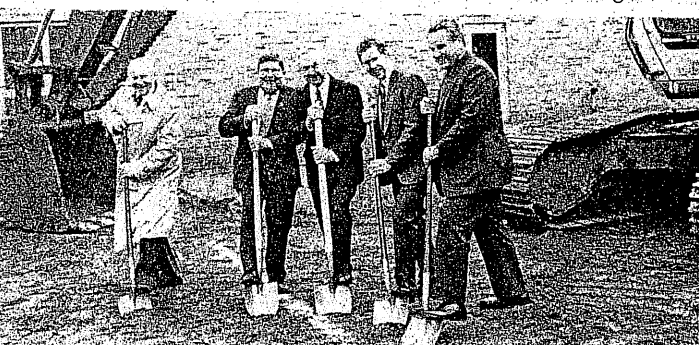
Groundbreaking for the skilled care Dujarie House addition and renovation: (l. to r.) Br. Thomas Shaughnessy, director of Dujarie House; Br. Richard Gilman, provincial counselor; Br. William Geenen, provincial; Vernon Feather, representative of The Troyer Group, architects and planners; and Jim Lusk, president of Verkler, Inc., general contractors.
