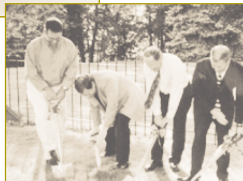
Ground Breaking for new addition to Dujarie House.
